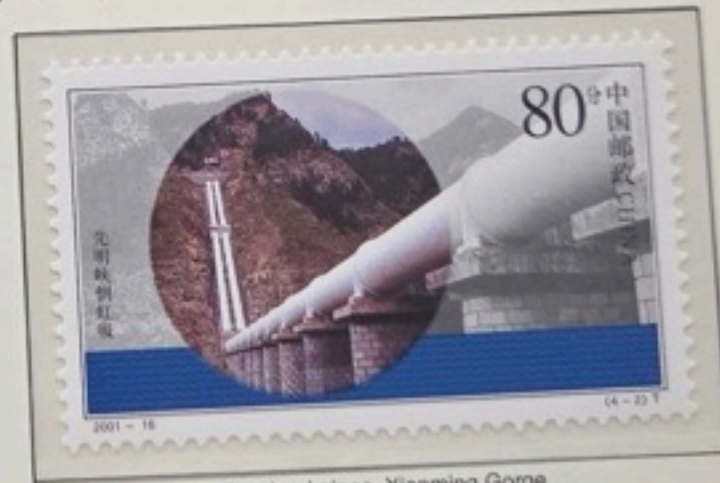
Overland pipes, Xianming Gorge
