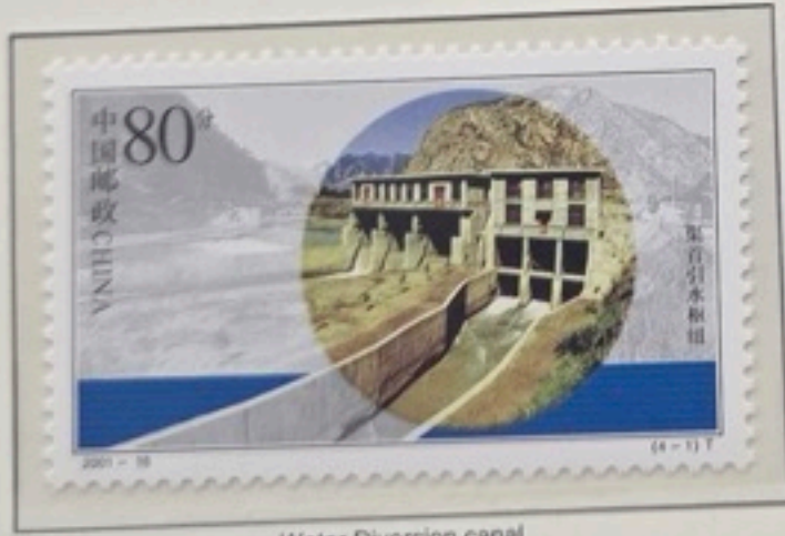
Water Diversion canal
